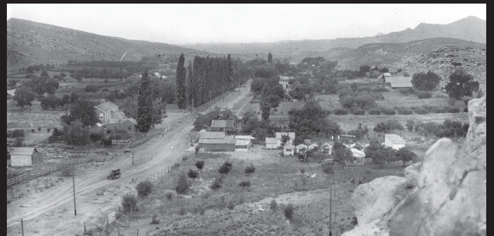
Looking south on Main Street in 1915. The schoolhouse is on the left, and the traveler's rest, the Log Cabin Inn, is on the right.
