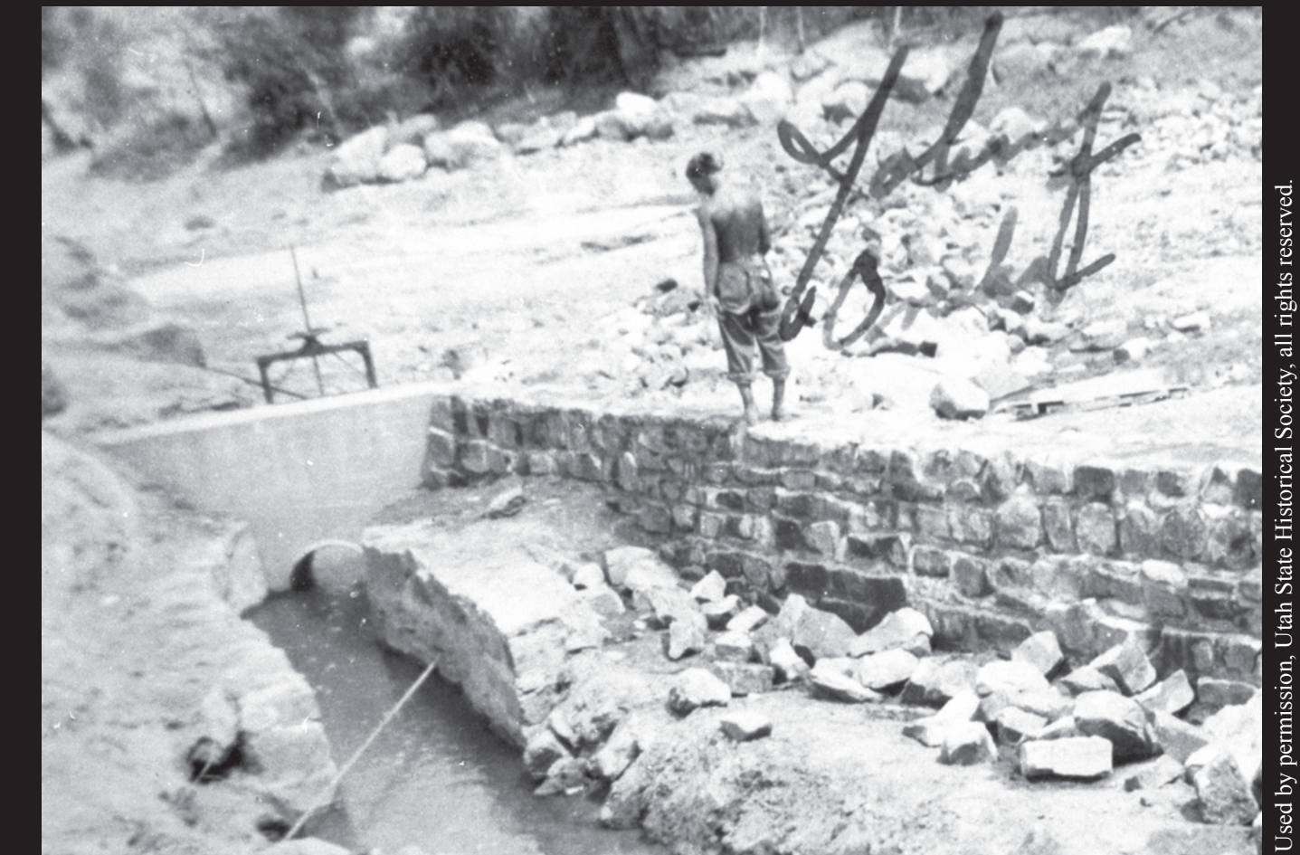
Jonny Onika, a CCC crew member, inspects a retaining wall. The crews also lined rivers with rocks, a process called “riprapping and cribbing,” to contain erosion and flooding.
